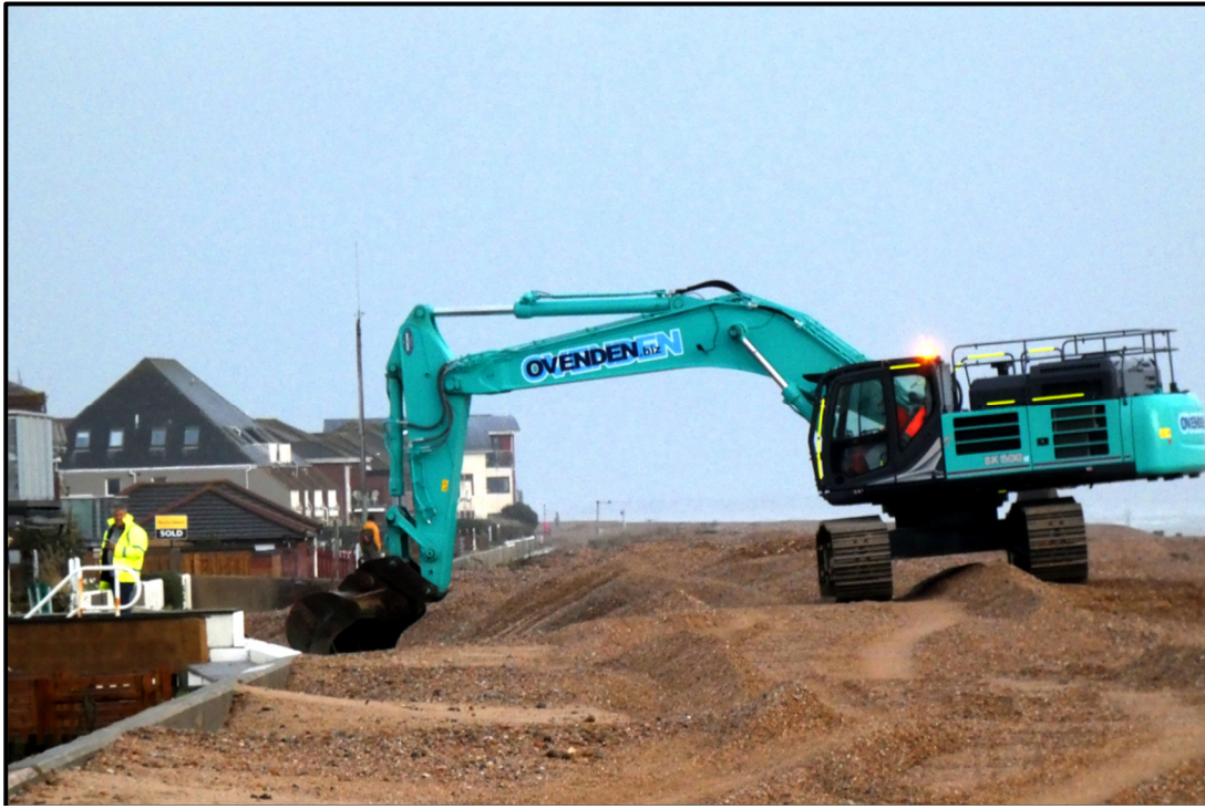
The Digger working at Eastoke to repair the barrier
