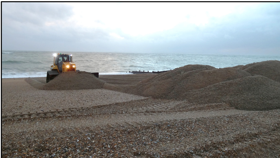
Bulldozer at Eastoke rebuilding the barrier
