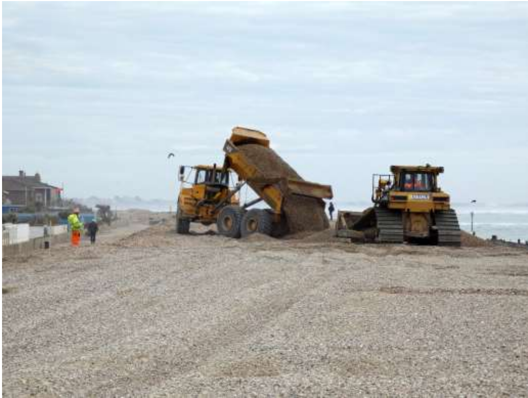
Pic 2: Showing the rectification works at Eastoke
